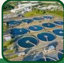
Raw Water Treatment
